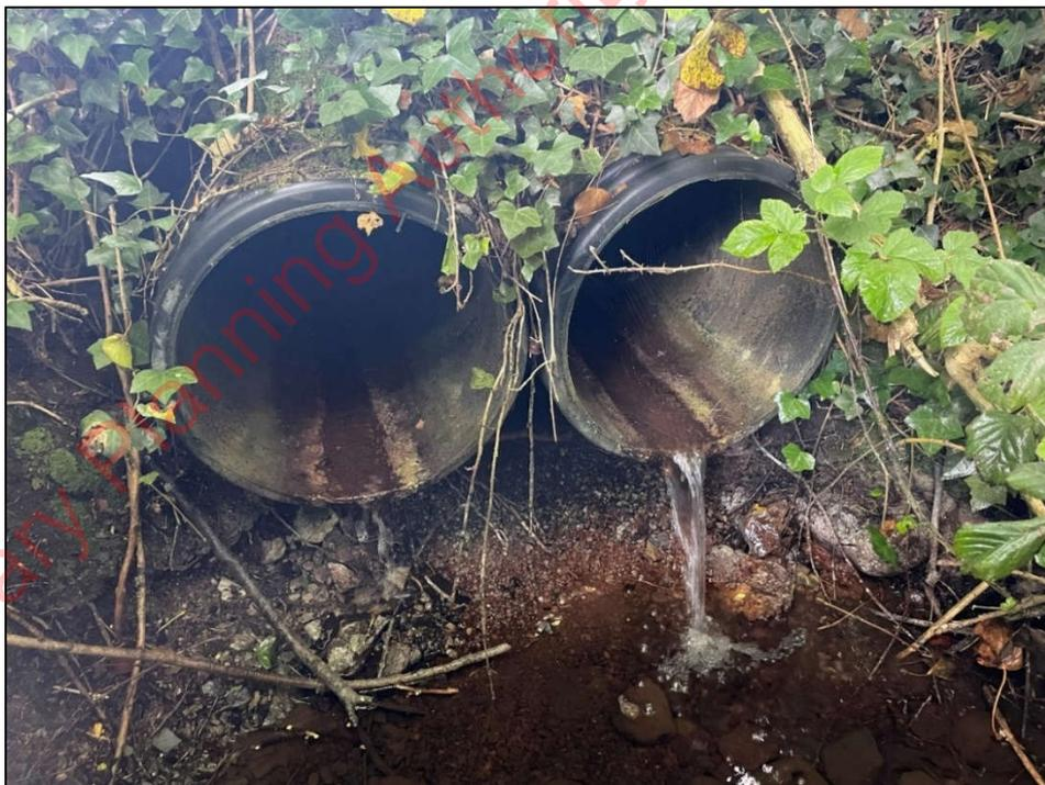
Plate 6-31 Double piped culvert at water crossing 4.
