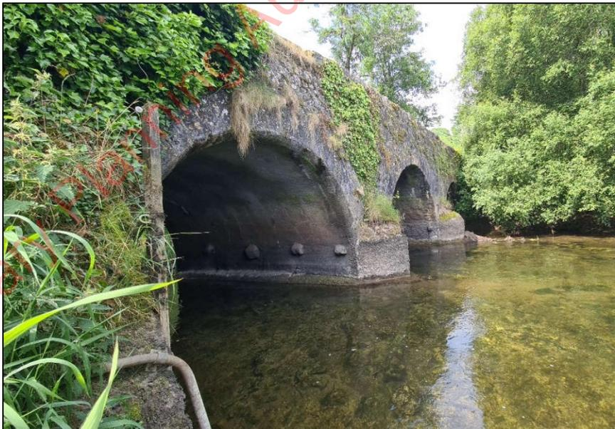
Plate 6-27 Triple stone arch with plaster underneath over crossing 2.
